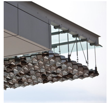
Detail of the suspension system
