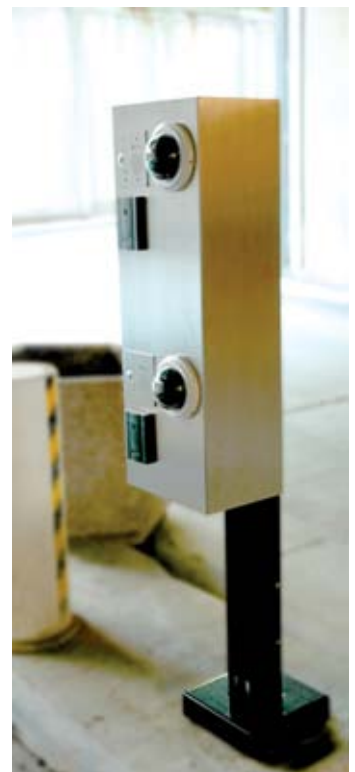
Security camera post & card access enclosure
