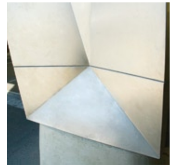
Concave forming of the cladding
