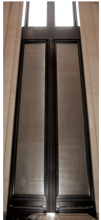
Custom stainless steel mesh louvers
