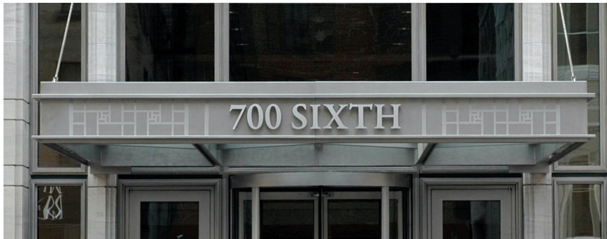
Exterior stainless steel canopy cladding
