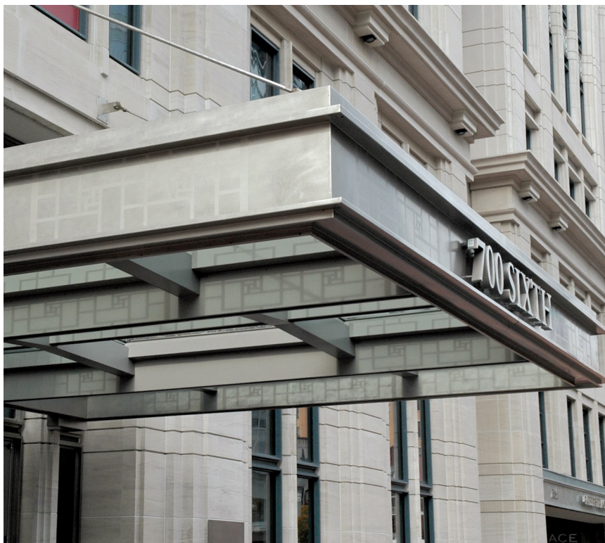
Stainless steel canopy cladding with etched pattern
