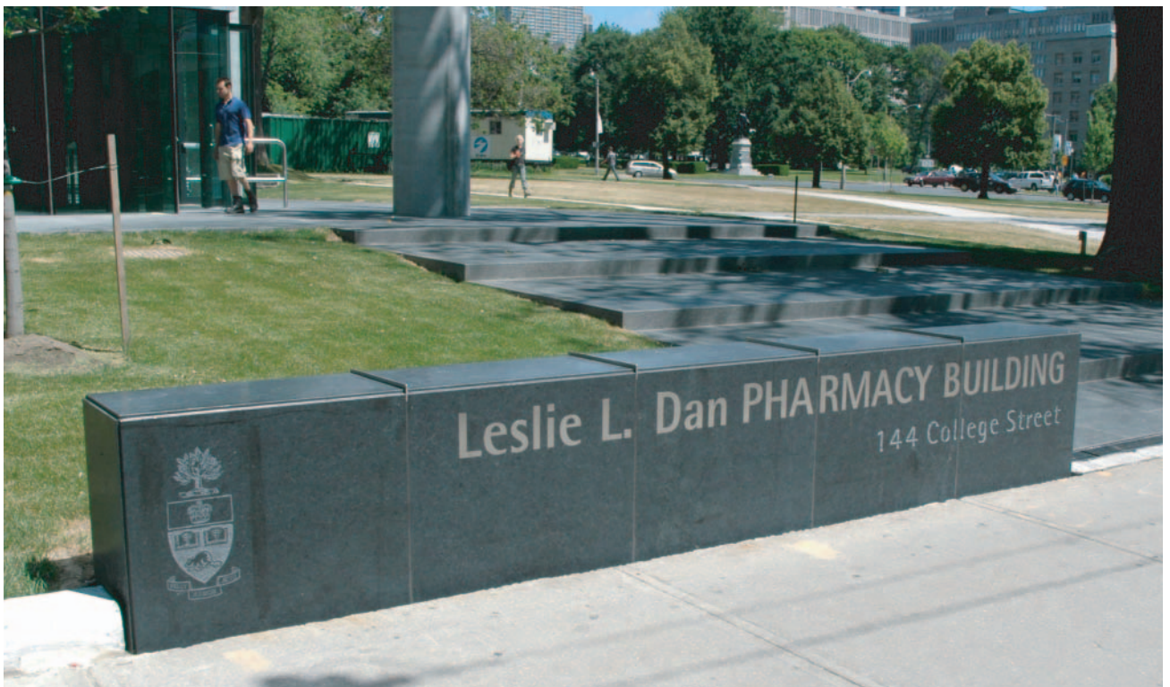
Precision carved granite and incised waterjet cut st. stl. lettering
