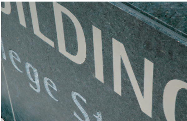
Waterjet cut, brushed st. stl. graphics incised into 1-1/4" thick granite
