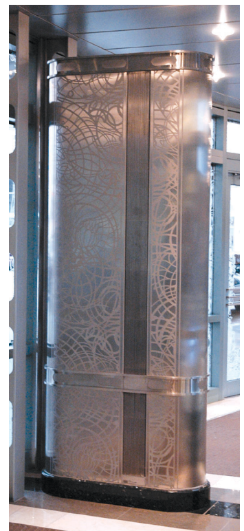
Custom stainless steel clad air supply tower
