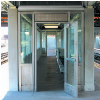
Cabins - approx. 9' wide by 60' long
