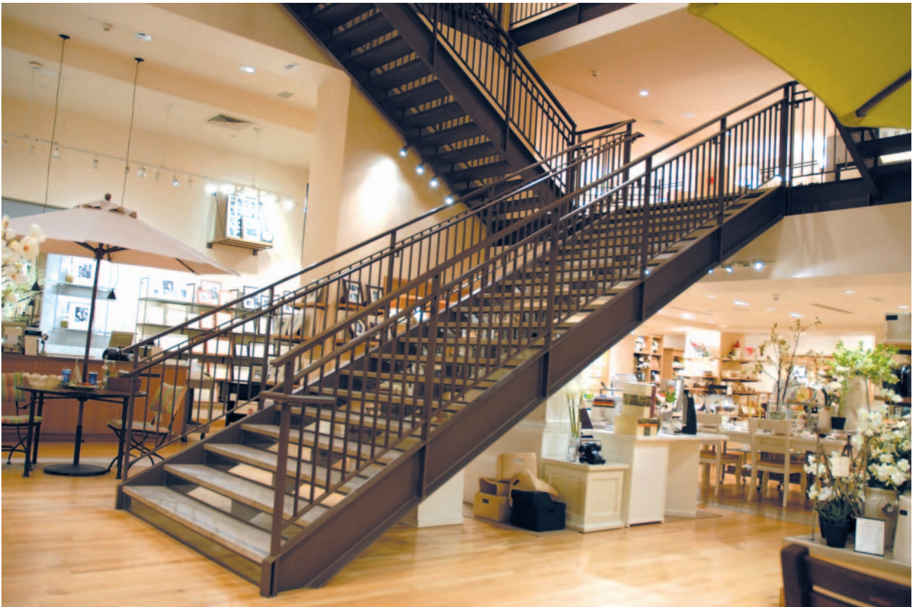
Painted steel staircases with concrete filled pan type treads and glass risers
