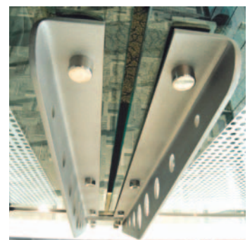
Custom stainless steel posts - shot blasted finish
