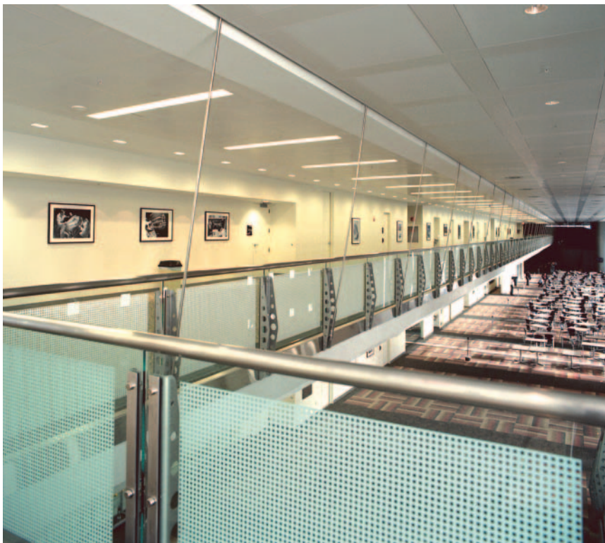
Cantilevered floor supported by stainless steel suspension rods
